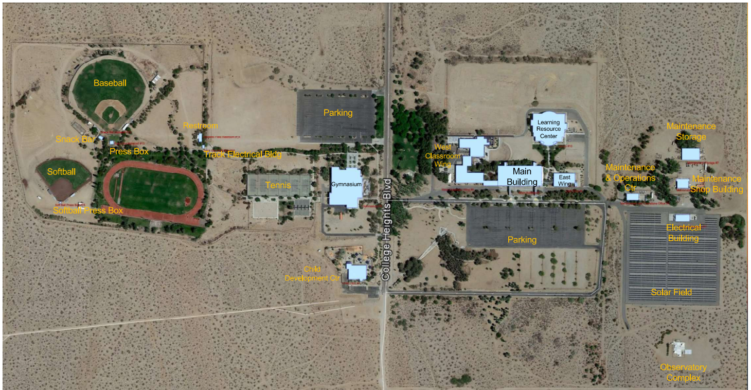
Figure 1: Aerial View of IWV/Ridgecrest Campus
