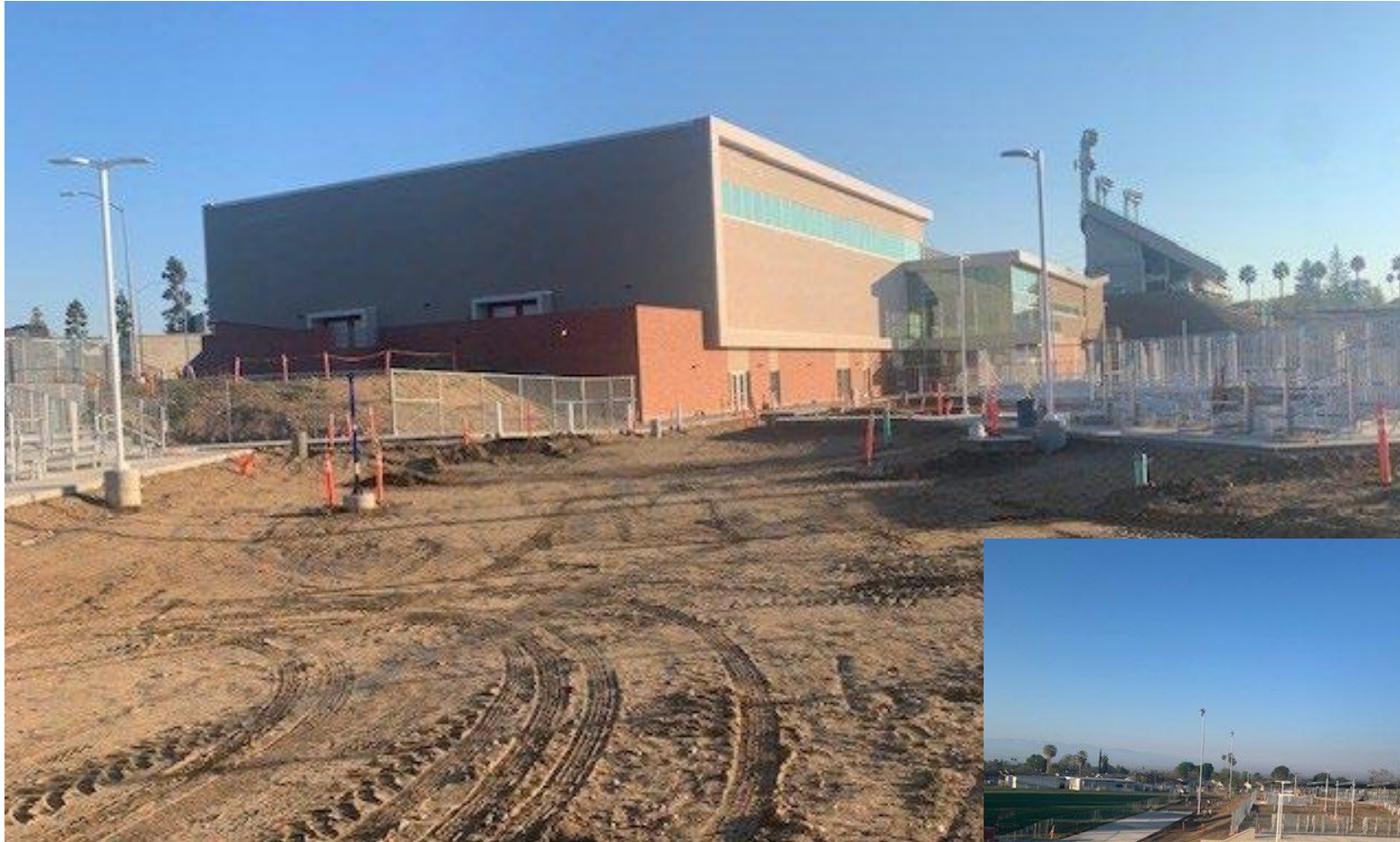
Renegade Athletic Complex Construction Complete December 2024
