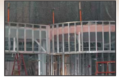
A view of the Student Center Remodel where the staircase was removed.
