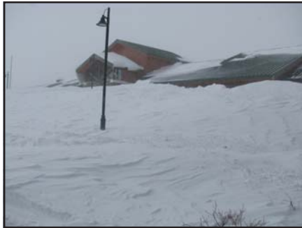
Front entrance to the Mammoth Lakes campus.
